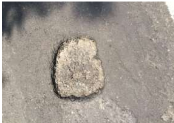
Gambar 7. lubang / potholes
