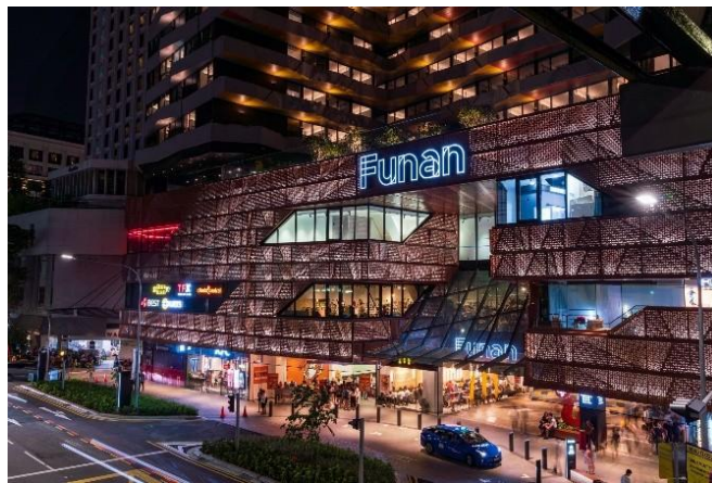
Gambar 2. 21 Fasad Funan Mall Sumber: https://cla.asia/project/funan-mall , 2018
