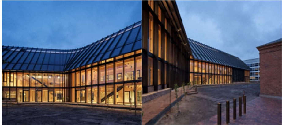
Gambar 2.10 Eksterior Center for Health, Copenhagen, Denmark
