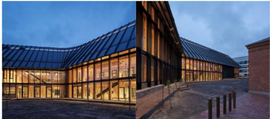
Gambar 2.10 Eksterior Center for Health, Copenhagen, Denmark
