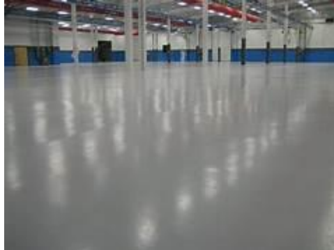
Gambar 18 Lantai Epoxy (Sumber: Google Images, 2025)
