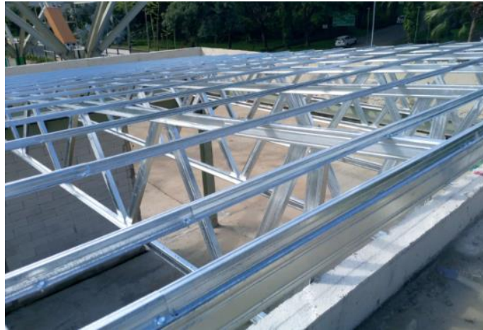
Gambar 4.33 Struktur atas lightweight steel frame (Sumber: Pinterest, 2026)
