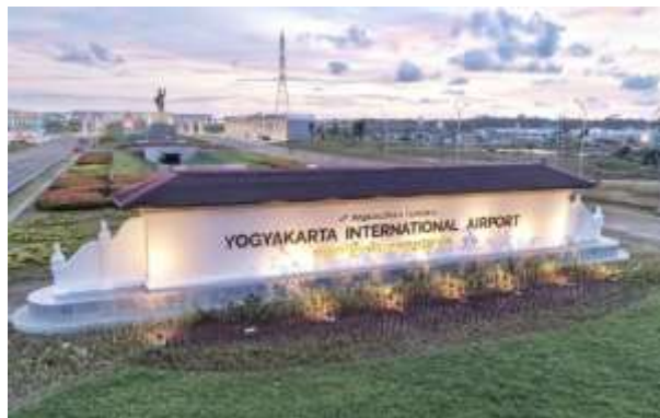
Gambar 2. 21 Yogyakarta International Airport
