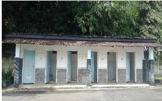
Gambar 104. Toilet Outdoor Lama
