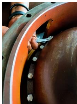
Gambar 17 pemasangan front cover
