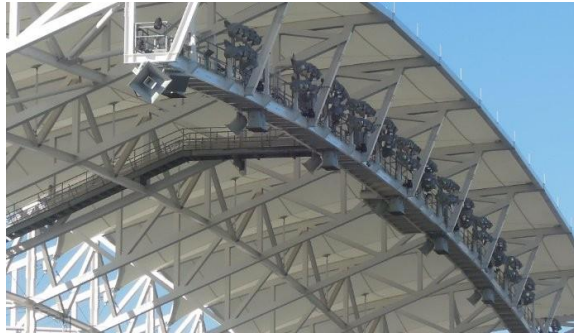
Gambar 9. Space truss (sumber: TensileInc,2016)
