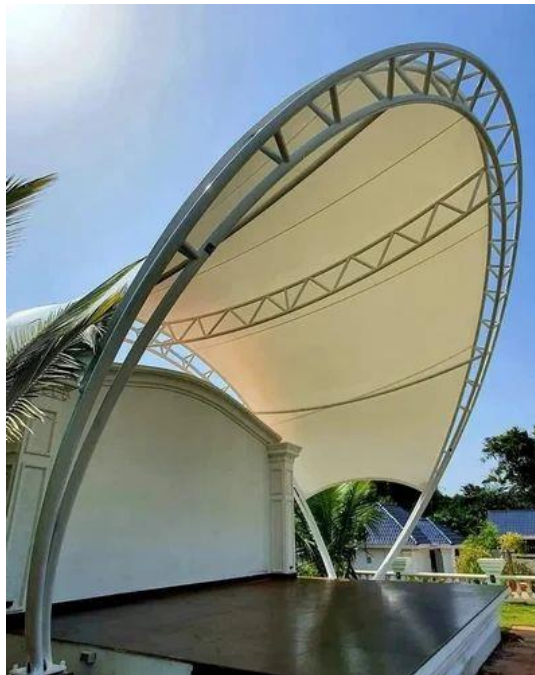
Gambar 10. Atap Membran (sumber: Design Fawz Tensile,2024)
