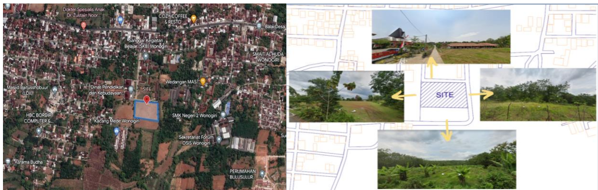
Gambar 1. Eksisting Site (Sumber: Google Earth, 2023)
