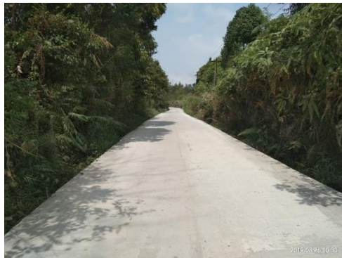
Gambar 4 Jalan cor ( https://wideazone.com , 2019)
