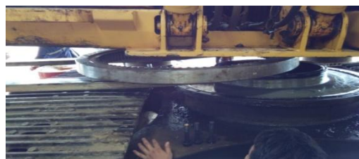
Gambar 4.5 Assembly Swing Circle Tahap 1
