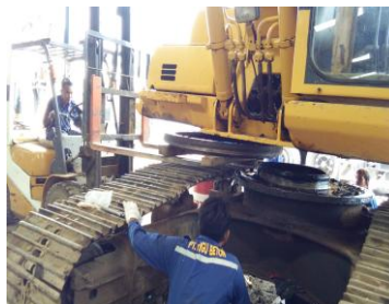
Gambar 12 Disassemble Swing Circle Tahap 6
