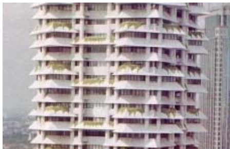
Gb. 55. Sirip-sirip kanopi Wisma Dharmala Sakti
