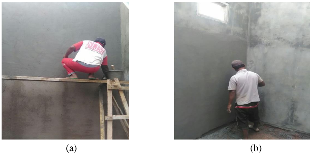
Figure 1. Plastering work (a) and Coating work (b)
