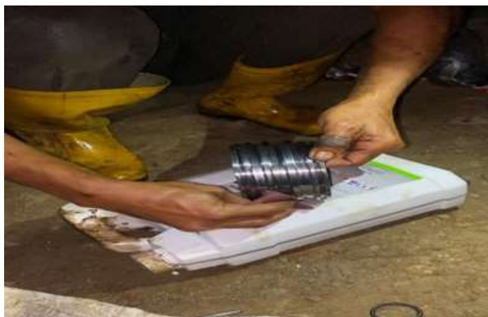
Gambar 5. Pencucian piston
