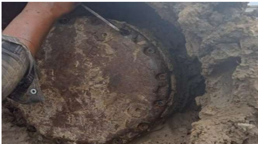
Gambar 14. Pemasangan Case Travel Reducer
