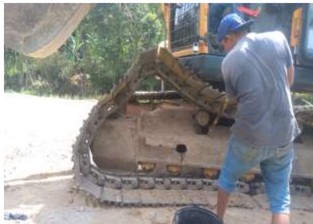
Gambar 21. proses pemasangan track shoe assembly
