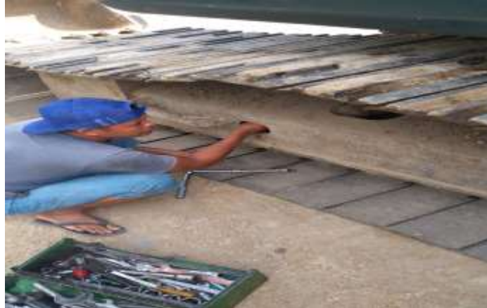
Gambar 22. proses pemasangan grease valve
